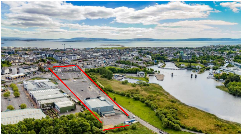
Phasing wrap Dyke Road
